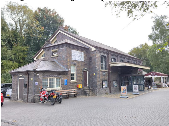
The Goods Shed - external aspect 4
