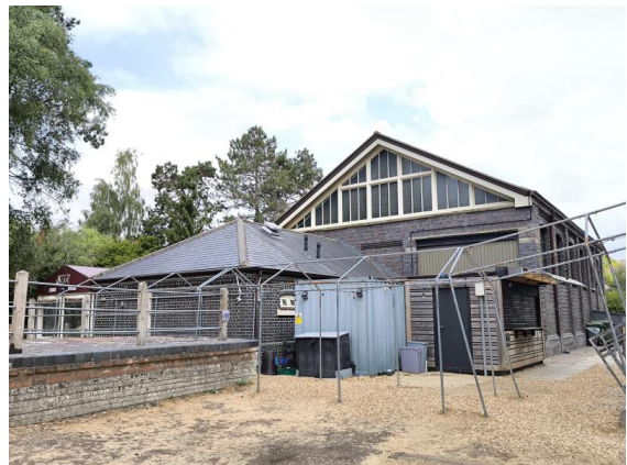
The Goods Shed - external aspect 3
