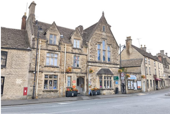
The Old Court House - West elevation
