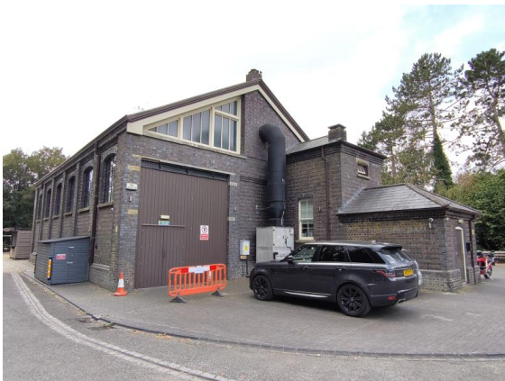
The Goods Shed - external aspect 2
