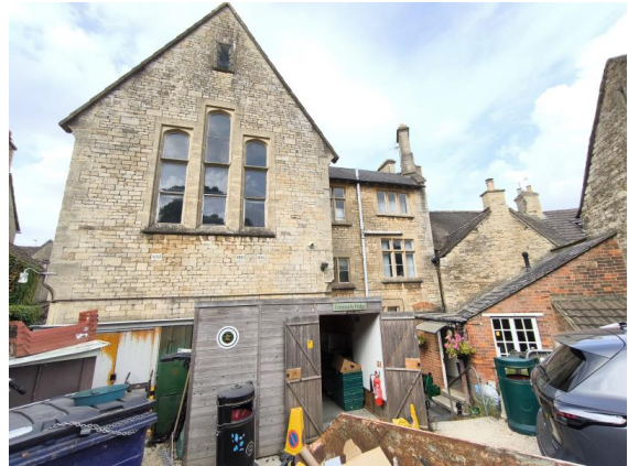
The Old Court House - East elevation
