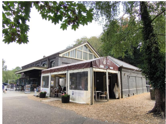
The Goods Shed - external aspect 1
