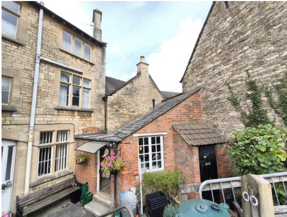
The Old Court House - rear extension
