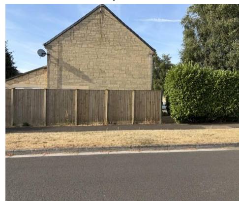
Site Four. Conyger Road before Bartley Croft
