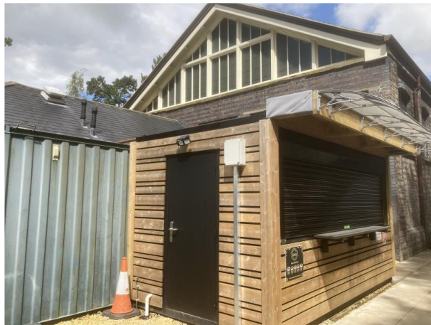
Storage Container and Bar area
